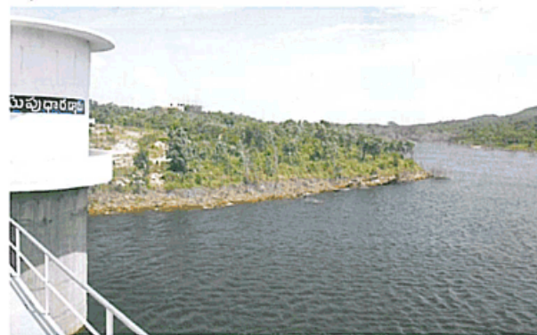
Papavinasanam Dam at Tirumala
